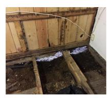
extremely frail wood, using a defective construction; there was no ridge beam, for example.
