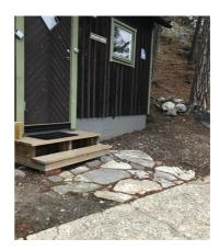
At some point after the military experiment was discontinued, a wooden terrace was constructed in front of one of the remaining buildings. To restore the 1940s exterior, the terrace was demolished along with the wooden walkways between the jetties. Below the planks we found concrete paths from the original seal station, which we carefully restored.
